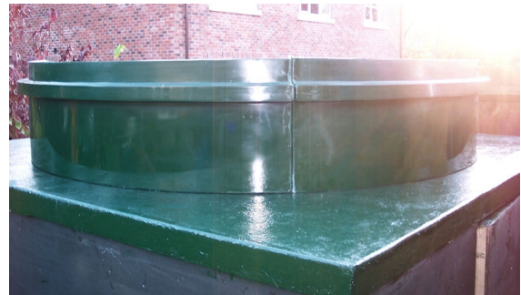
The track fitted to a flat-roofed shed
