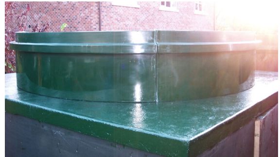
The track fitted to a flat-roofed shed
