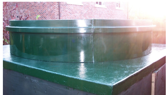
The track fitted to a flat-roofed shed
